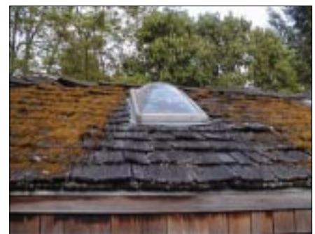
Galvanized flashing around this skylight releases zinc into rainwater and prevents moss from growing below it. (Photo by Bruce McCune)
